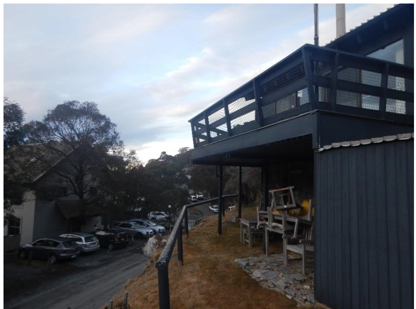
Figure 7 : Photo of the existing deck to be reconfigured
