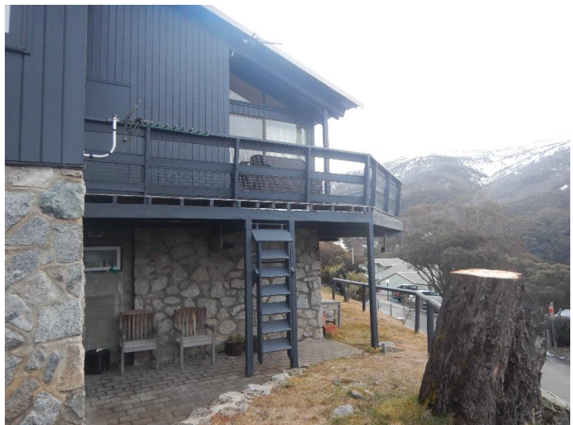
Figure 8: Photo of the existing side deck to be removed and location of proposed additions
